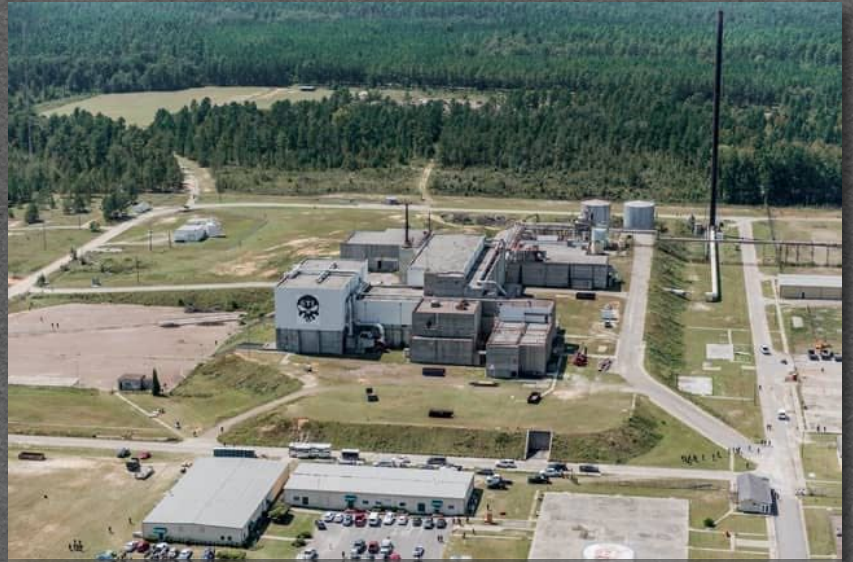
# GTI Training Facility in Barnwell, SC
