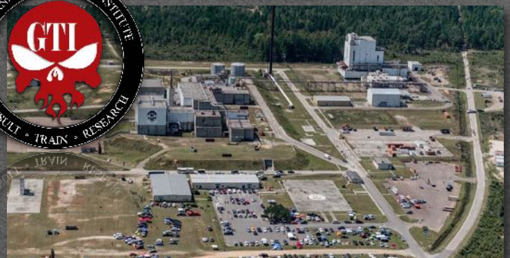
GTI Joint Operations Center in Barnwell
